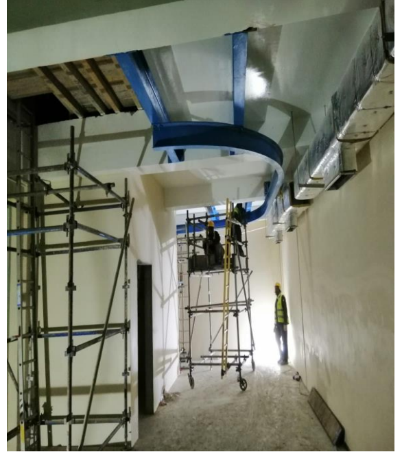
Structural Works / Ducting – Shuaibah III Expn II Diesel Plant (2019)
