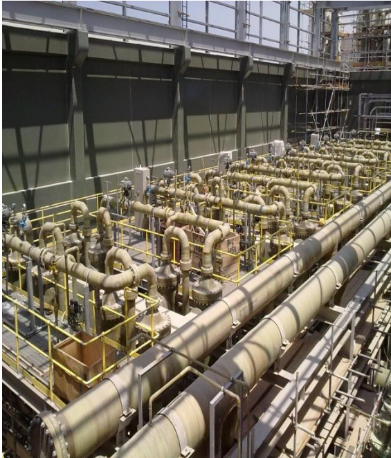
GRP Piping works – Rabigh Power Plant (2012- 2013)
