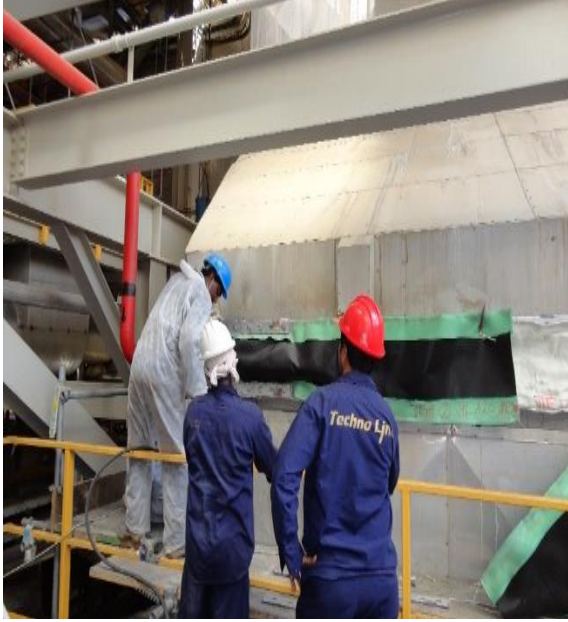
Replacement of Fabric Expansion Joints, SWEC-IWPP, Shuaibah-Jeddah (2013 – 2014)
