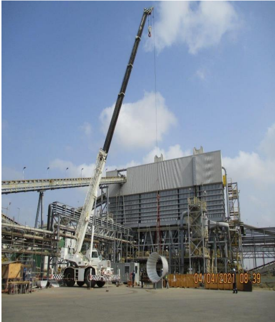
Mechanical/Electrical/Instrumentation Works for Furnace-1 Modification at ILMENITE SMELTING PLANT AMIC – JAZAN (2019-2021)
