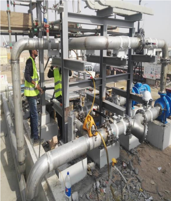
Stainless Steel Piping Works – Shuaibah III Expn II Diesel Plant (2019)
