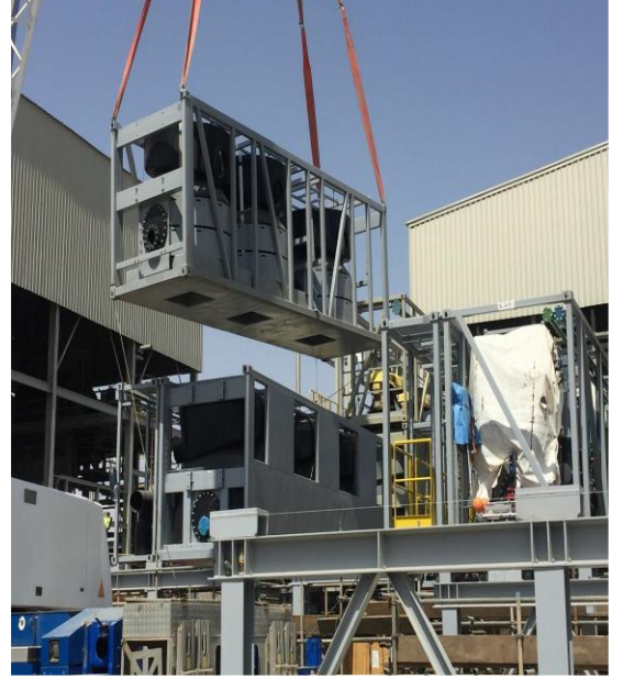
Installation of Mechanical Equipment, Ma'aden Goldmine , Al-Amar (2017)
