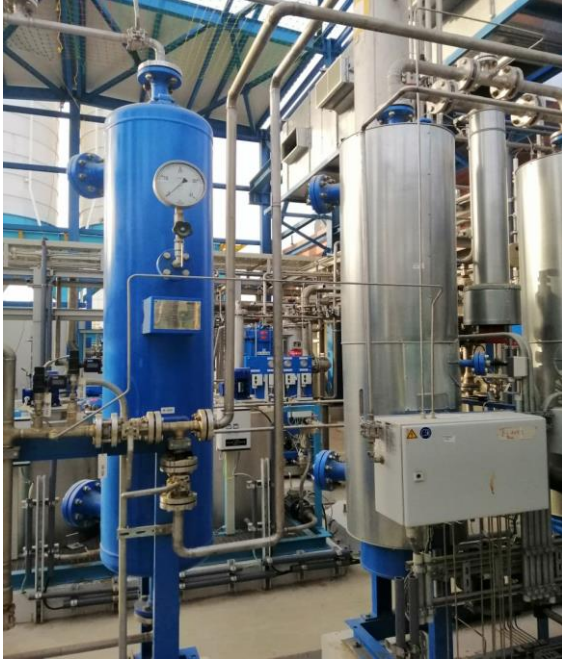
Co2 Piping / Tanks Works – Shuaibah III Expn II Diesel Plant (2019)
