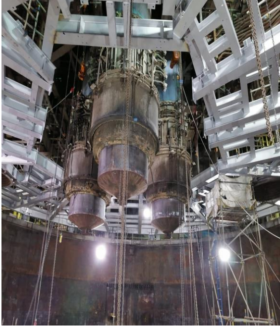
Furnace Modification Works – ILMENITE SMELTING PLANT AMIC – JAZAN (2019-2021)
