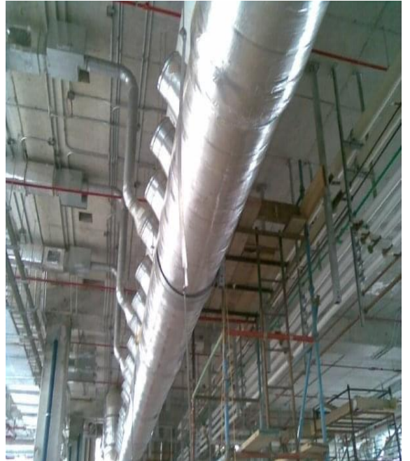
MEP Network Installation Works – KAUST Project Tuwal (2008)
